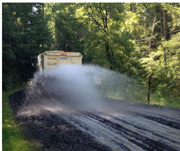
**Figure 27.** Adding water to a dry road surface.
