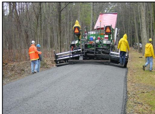
**Figure 15.** Paver placement of DSA with proper crown.
