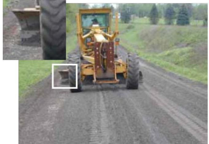
**Figure 31.** Grader grooming the road. Notice the grader blade is not carrying a lot of material.
