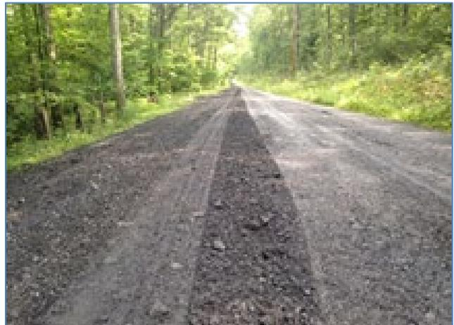
**Figure 32.** Before & after first pass of 10-ton roller.
