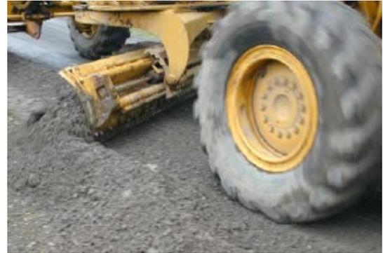
**Figure 24:** Wet material rolling off blade.
