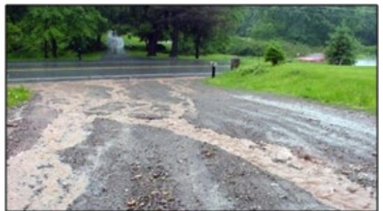
Figure 19. Water in wheel tracks.
